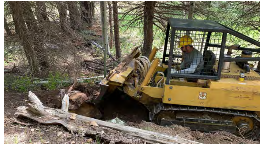
IMAGE 12. Mechanized trail construction 5
